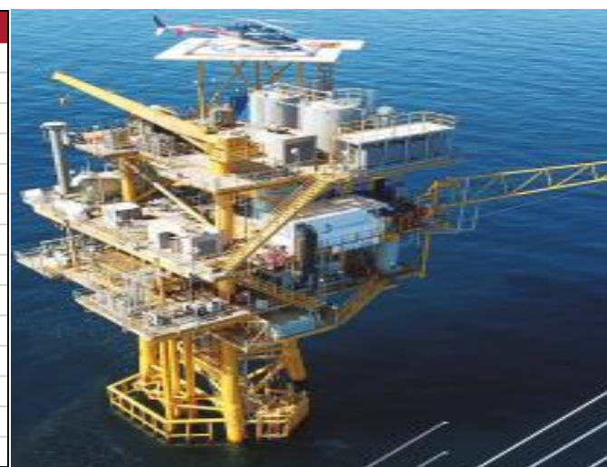
Figure 13: SM71 platform, key infrastructure with ullage
